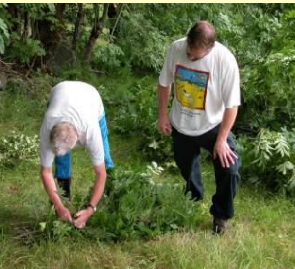
A 1m long birch twig is used to tie the bundle together
